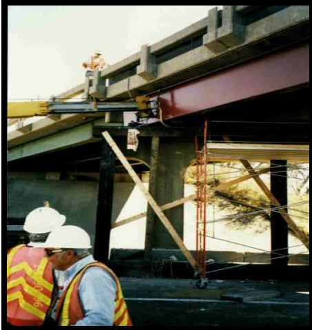
Bridge "Jacking" and Replacing Steel Girder
