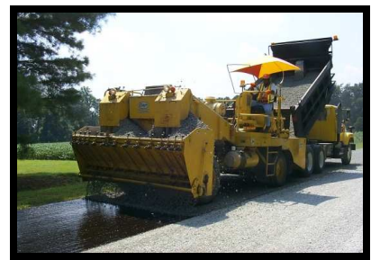
Retreatment (Chip Sealing) Operation
