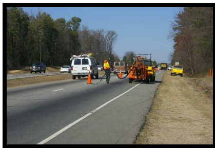
Crack Sealing Operation
