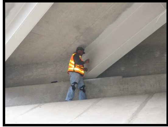
Freshly Painted Steel Bridge Girders
