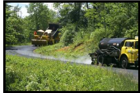
Pavement Preservation Bituminous Surface Treatment
