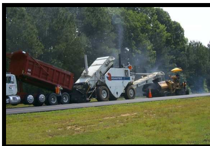
Contract Resurfacing Operation
