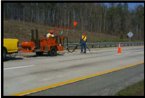
Pavement Preservation Crack Sealing
