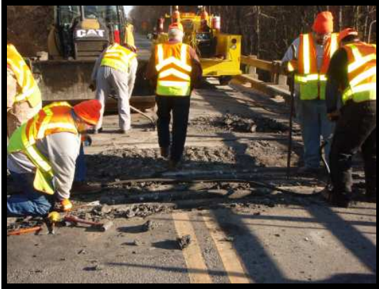
Replacing Expansion Joint
