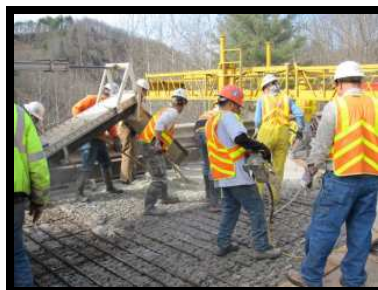
Bridge Deck Overlay Operation
