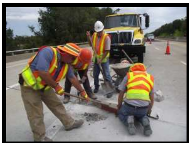
Bridge Deck Joint Repair Operation
