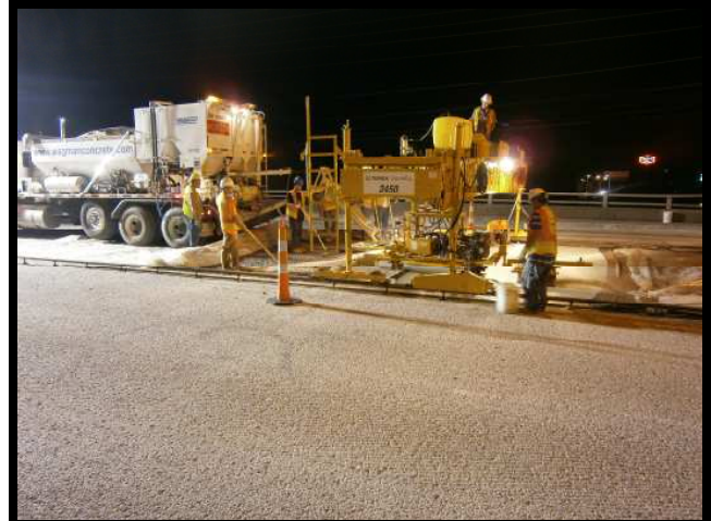
Replacing Concrete Deck
